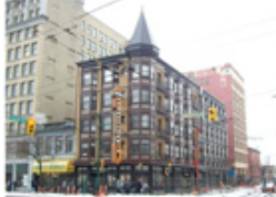
Pennsylvania Hotel, 412 Carrall Street
