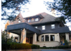
Greencroft, 3838 Cypress Street
